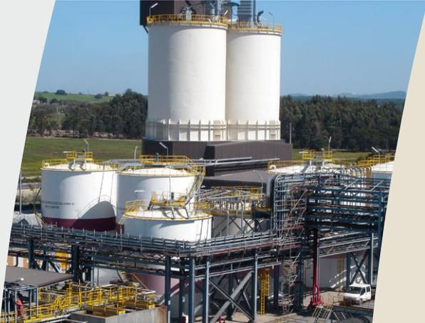
As a result of increasing environmental protection regulations, Flue Gas Desulphurisation (FGD) Plants have been installed on power plants worldwide since the early 1980's. The predominant technology utilised is based on wet scrubbing which produces widely varying corrosive environments within the process equipment and flue gas ducting. Such an FGD Plant may require more than 4 different types of corrosion protection systems (see typical fields of application).
